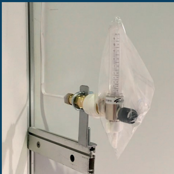
Oxygen points are being installed to cater for 400 seriously ill patients.
